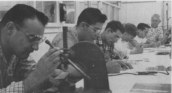
ASSEMBLY OPERATION, attaching small electronic components to the printed circuit cards, is done with care and patience. Cleanliness is a necessity as any foreign matter in the assembly
